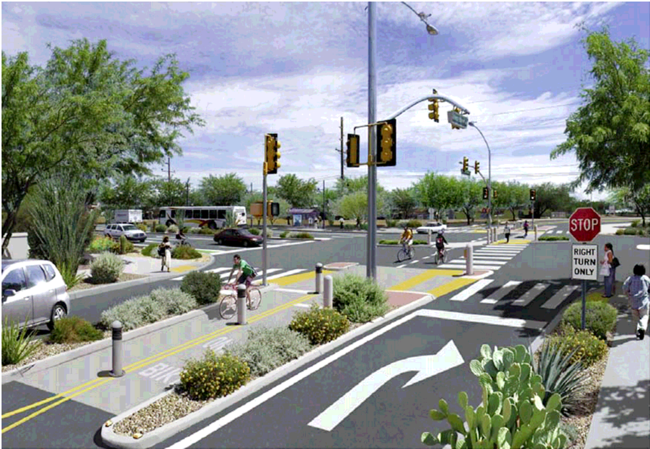
Proposed bicycle/pedestrian signal to be installed at Treat Avenue and Grant Road, as part of the Grant Road Improvement Project. The TOUCAN style signal prioritizes bicycles and pedestrians and helps reduce car traffic along Treat.. Tucson currently has four TOUCAN signals in use.
