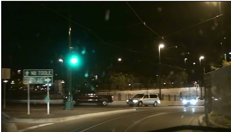
Figure 5: View of Raised Island at Night
