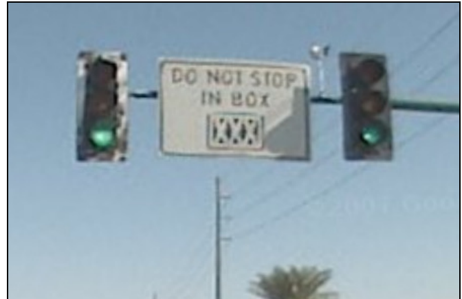
Figure 10: Pavement markings and signing to discourage blocking of intersection by vehicles
