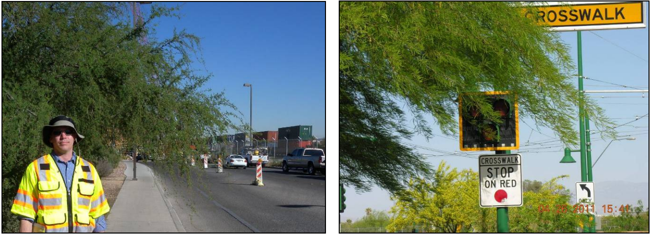
Figure 16: Tree Branches Blocking Sidewalk and Blocking View of HAWK Beacon
