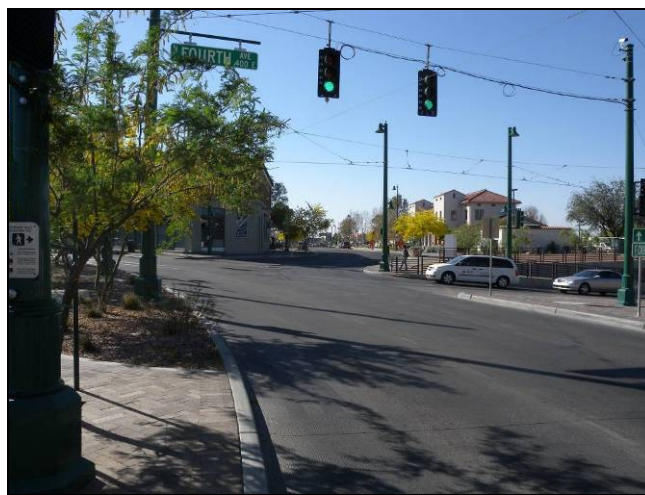
Figure 4: Pavement Markings Difficult to See During the Day
